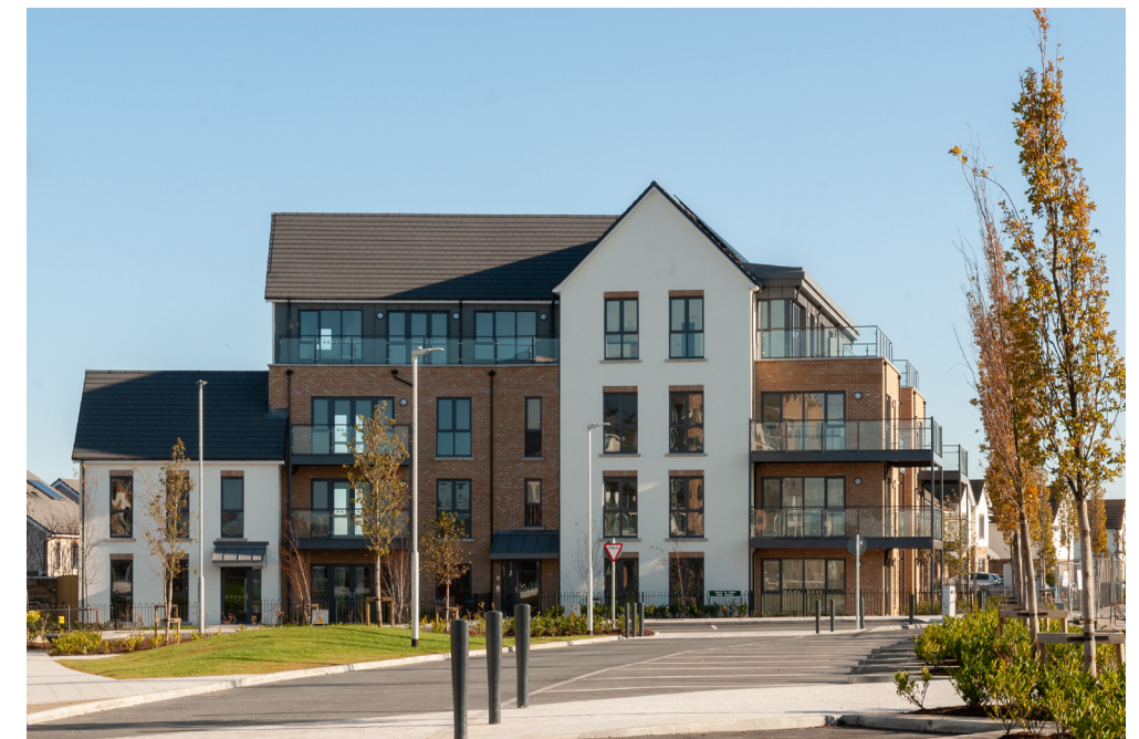
Below: A Gannon Properties development of 14 social housing units, provided as Part V, + creche on Miller's Square, Park Avenue
