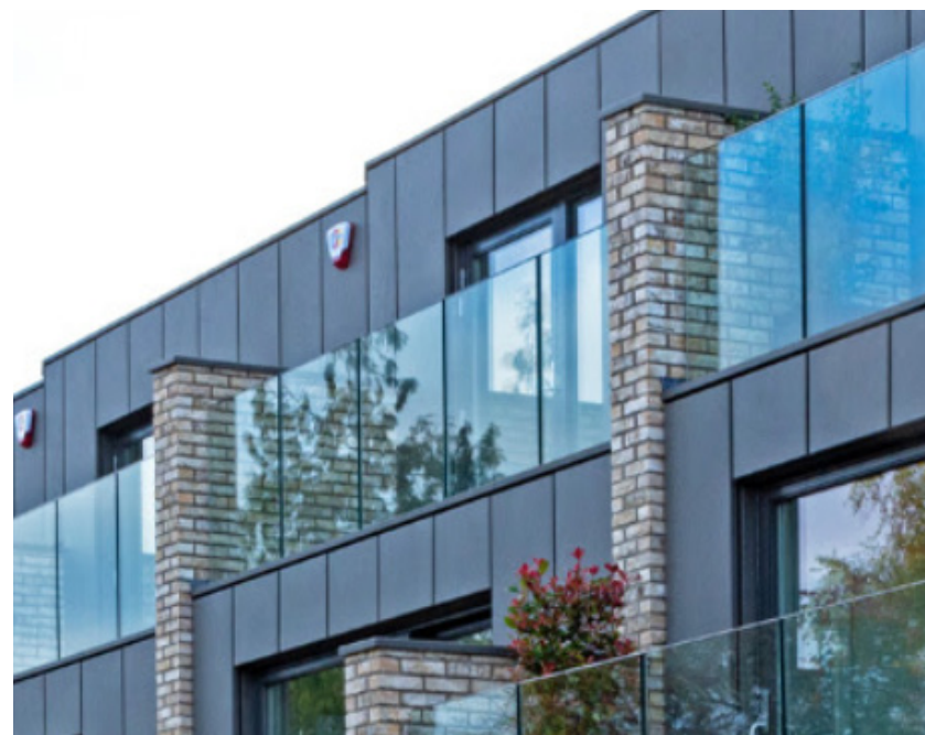
Glass guarding at balconies to apartment blocks
