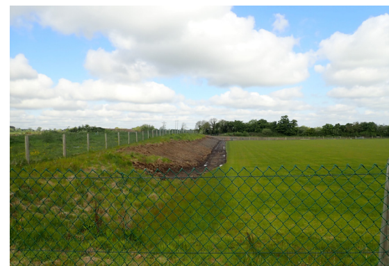
Left: Townland boundary to northern boundary of the site on the left, new playing pitch on the right
