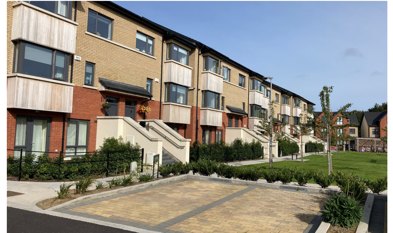
Above: Example of well landscaped surface car parking
