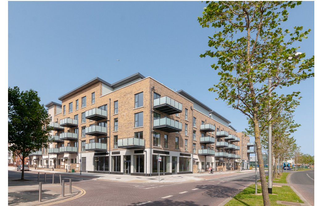
Above: Gannon Properties development of 84 social housing units + mixed-uses provided as Part V in Clongriffin
