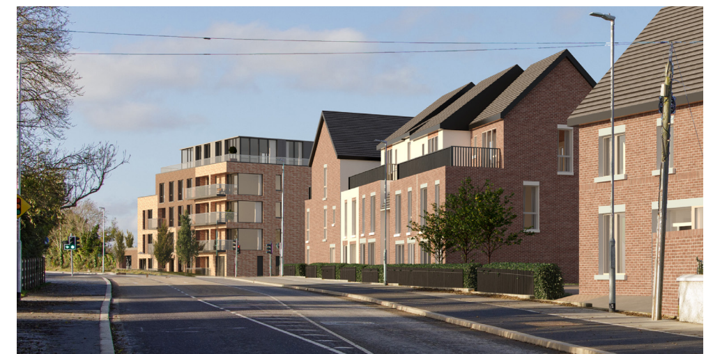
Above: Increased building height onto Rathbeale Road (CGI and verified view by Modelworks)
